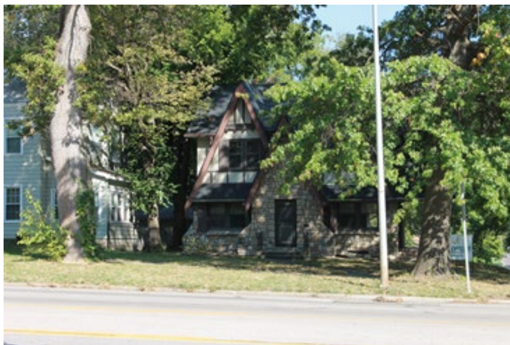
Figure 22: showing high style Tudor Revival house at 1400 West Broadway Boulevard, by Chalfant
