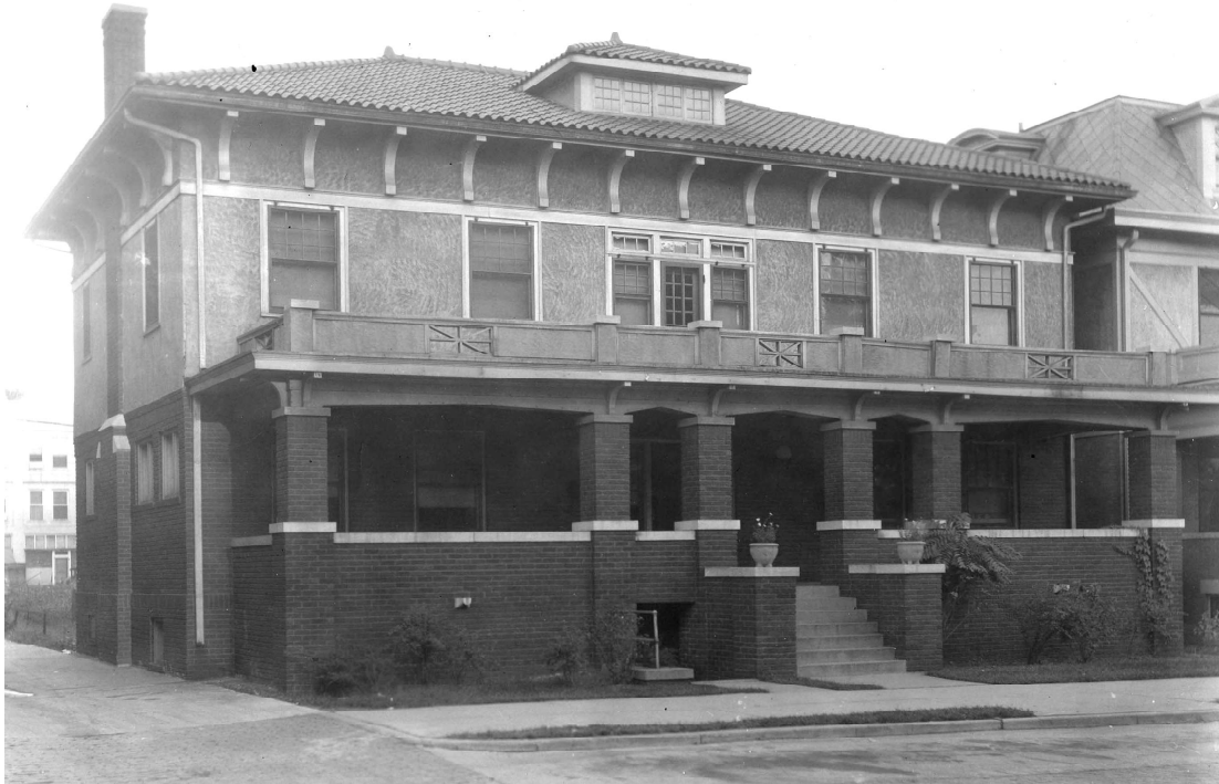
Image F Sojourners Club, West Façade, c. 1928. Note the original configuration of the veranda and second story terrace (closed balustrade) as well as the contrasting paint on the second story stucco and wood. (Truman State University).
