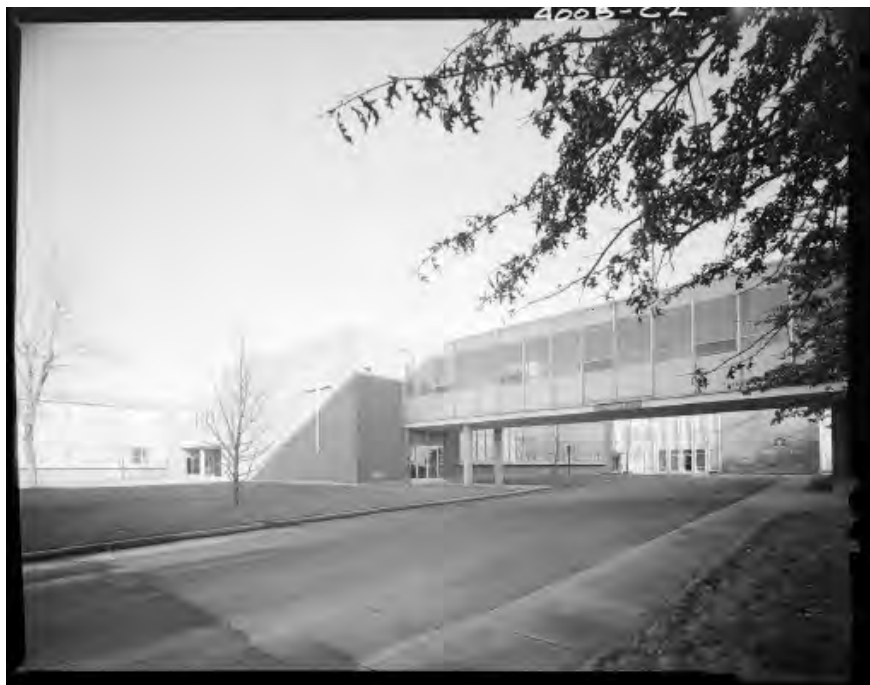
Figure 10. Notre Dame College Buildings in December 1970. Source: Henry T. Mizuki, photographer, Missouri Historical Society, Photographs and Prints Collection, Mac Mizuki Photography Studio Collection, id: P0374-04005A.
