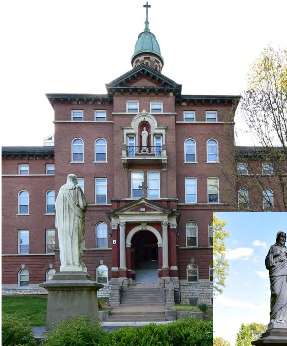
Figure 8. Detail of Chapel wing entrance on the east elevation of the Motherhouse. The Statue of the Sacred Heart (1952) faces the building. Source: Brad Finch, April 2021.
