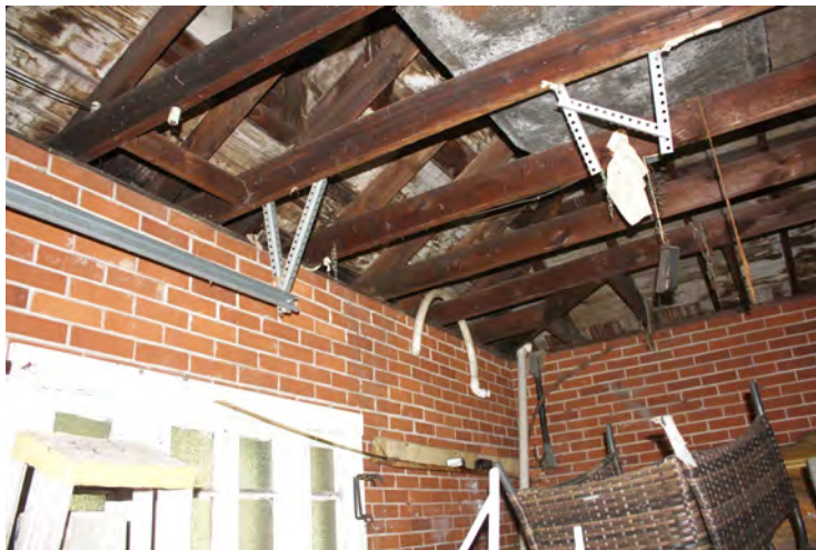
Figure 36. Garage interior. Left: Curving roof trusses. Right: doorbell ringer attached to roof truss. Photos by Homegrown Studio and Louis Murray, 2022.
