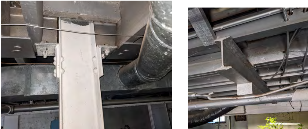
Figure 37. Basement ceiling structure. Photos by Homegrown Studio, 2022.
