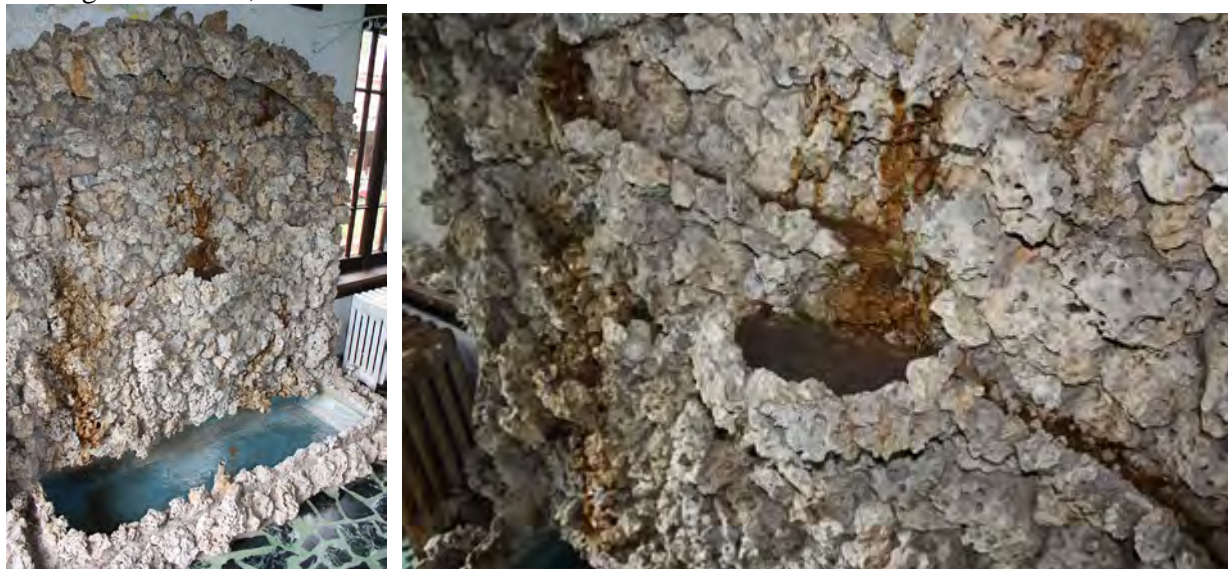
Figure 29. Interior Details, #1 Fairway. Sunroom/solarium fountain in operation. Photos by Homegrown Studio, 2022.
