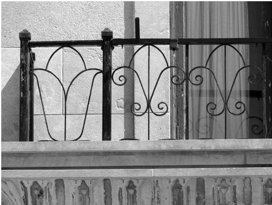
Figure C Detail of main entrance balustrade
