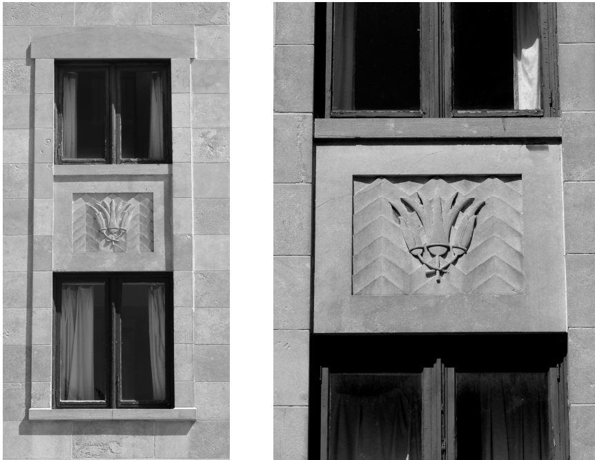
Figure D Detail of fenestration and spandrel on south (Harrison Street) façade.
