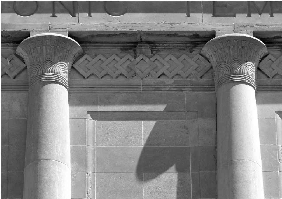
Figure F Detail of broken frieze and engaged columns on south (Harrison Street) façade.
