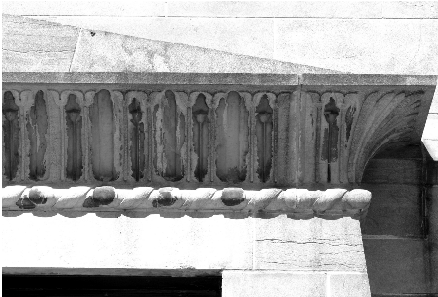
Figure I Detail of cornice for funeral door on east (High Street) façade.
