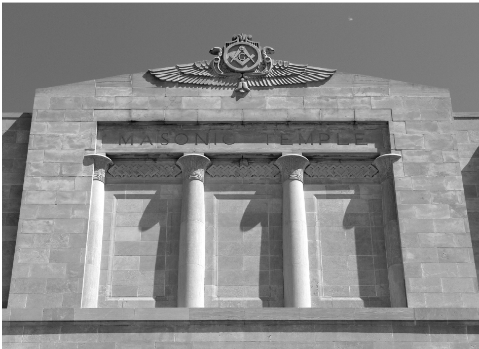
Figure E Detail of temple front on south (Harrison Street) façade.
