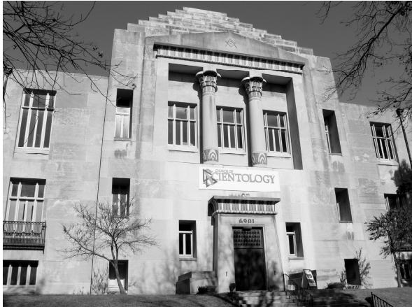
Figure DD Anchor Masonic Temple (1925). University City, Missouri. (Preparer's Photograph)
