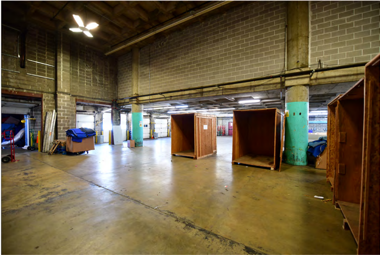
Figure 10. West loading bay area in the 1962 addition, looking NW. Source: Brad Finch, November 2022 (F10 on Photo Map 2).
