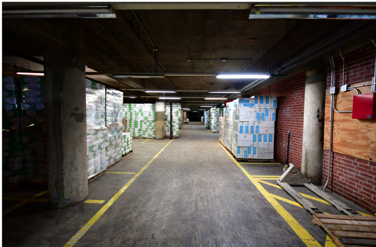
Figure 37. Fifth floor of 1946 addition, looking east. Source: Brad Finch, November 2022 (F37 on Photo Map 6).
