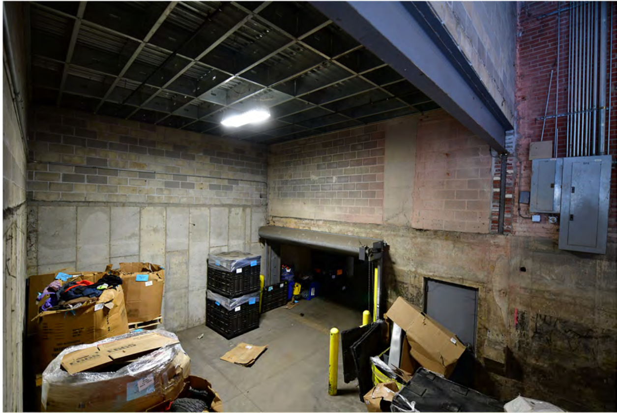
Figure 16. Location of former west paint rooms converted to basement access, looking NW. Source: Brad Finch, November 2002 (F16 on Photo Map 2).
