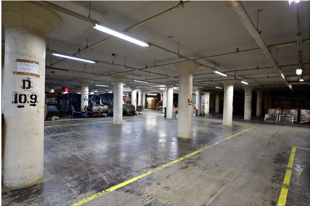
Figure 35. Third floor of the 1946 addition, looking southwest. Source: Brad Finch, November 2022 (F35 on Photo Map 4).
