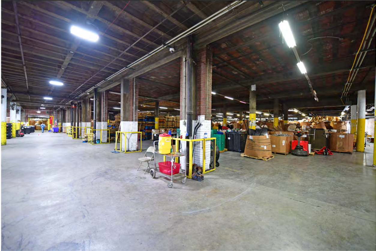
Figure 14. West addition to south dock, first floor, looking NE. Source: Brad Finch, November 2022 (F14 on Photo Map 2).
