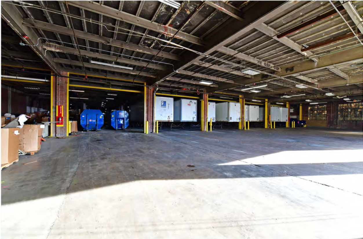
Figure 15. West loading dock addition, looking ESE. Source: Brad Finch, November 2022 (F15 on Photo Map 2).
