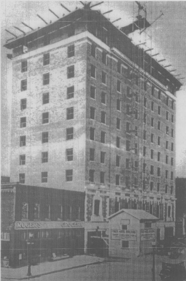
Figure Six. Construction of the Tiger Hotel, note the remodeled façade on the grocery store to the left.
