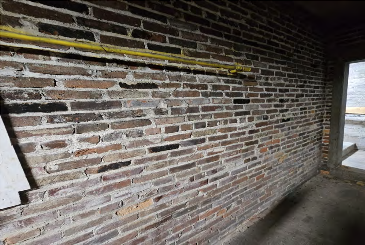
Figure 21: Boiler Room wall showing recycled bricks, basement, facing west
