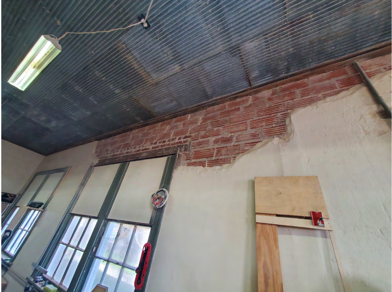
Figure 19: Close up of historic plaster, non-historic tin ceiling and historic wall
