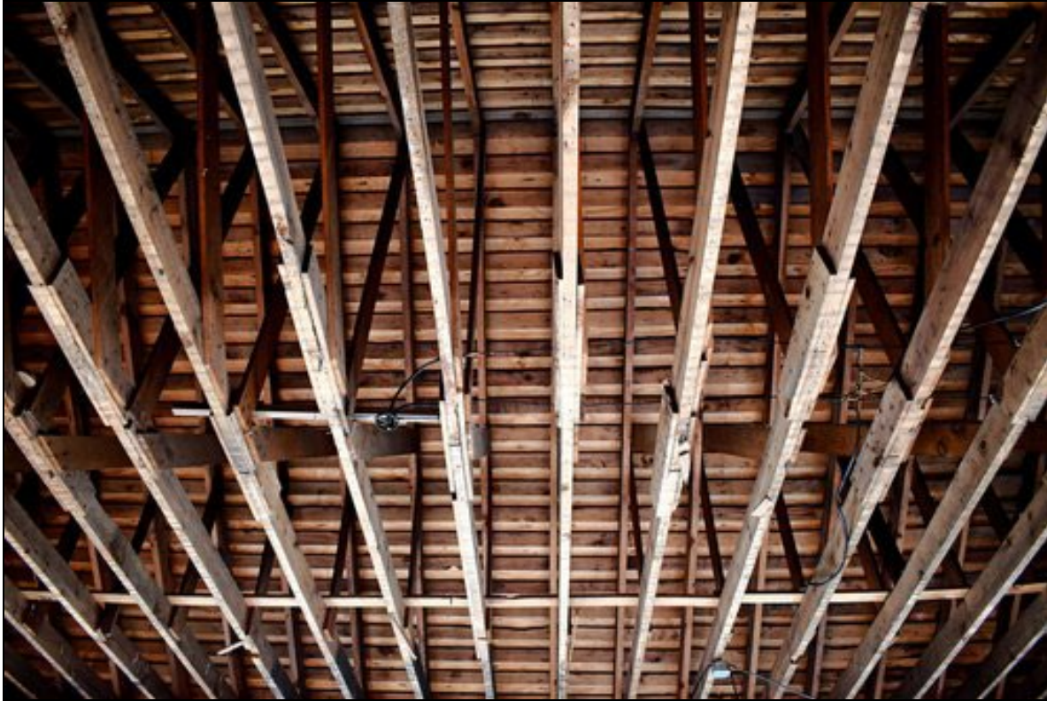
Figure 7. Exposed framing of the roof before renovation. McConnell, “Lincoln School...to become cultural center,” accessed June, 2024.
