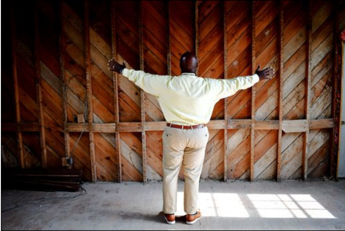
Figure 6. Exposed framing of the north wall before renovation. McConnell, "Lincoln School...to become cultural center," accessed June, 2024.
