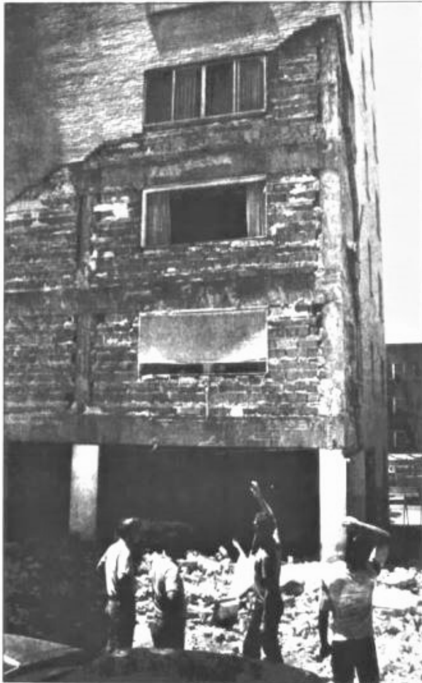
Figure 9. 1984 Image of Damage to the Northeast Corner of Sunset Tower. (Helliker, Kevin. "Brick Fall from Walls of Apartment Building; No Injuries reported." The Kansas City Times . May 14, 1984, 13. Newspapers.com.)
