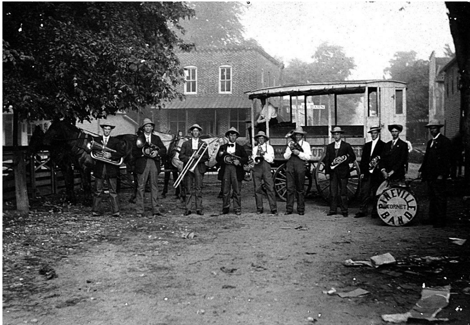
Figure 9: Cornet Band Ca. 1910 (in street east of courtyard)
