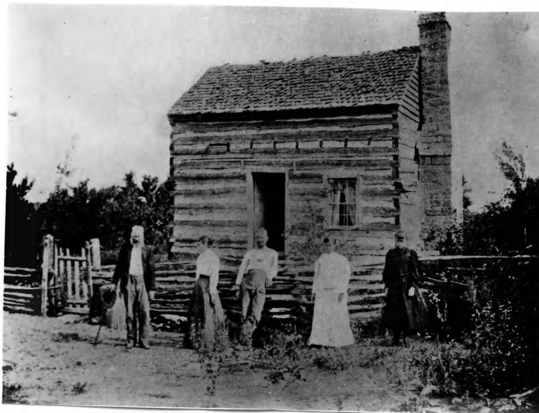
"Classic" Miller County Scotch-Irish single cell pioneer houseplace c. late nineteenth century. Fine squared logs with square notching, fine finished chinking, roofing, weather boarded gables, six-over-six sash, floored loft, finished stone chimney with drip cap. Split rail fencing with finished gate.
