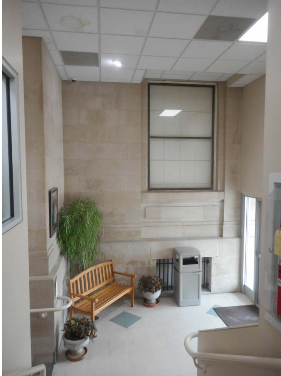
Figure 13: North segment of original east elevation exposed inside addition's north foyer, Stephanie Patterson, February 2022.
