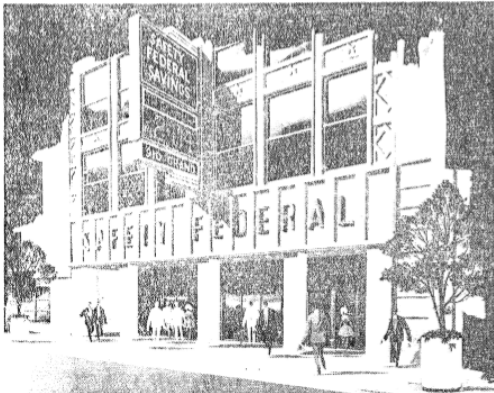
PRECAST CONCRETE PANELS and a new 6½-foot setback are features of facade changes in progress at the Safety Federal Savings and Loan association's building at 910 Grand avenue. Voskamp, Slezak & Jameson are architects for the project, scheduled to be completed in about 60 days.
