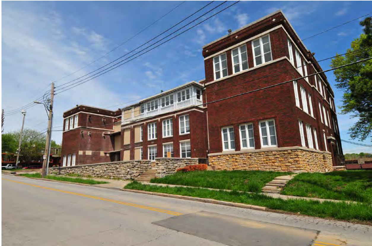
Figure 28. Swinney School, primary elevation showing the enclosed Open Air classroom. Source: Brad Finch, 2013.
