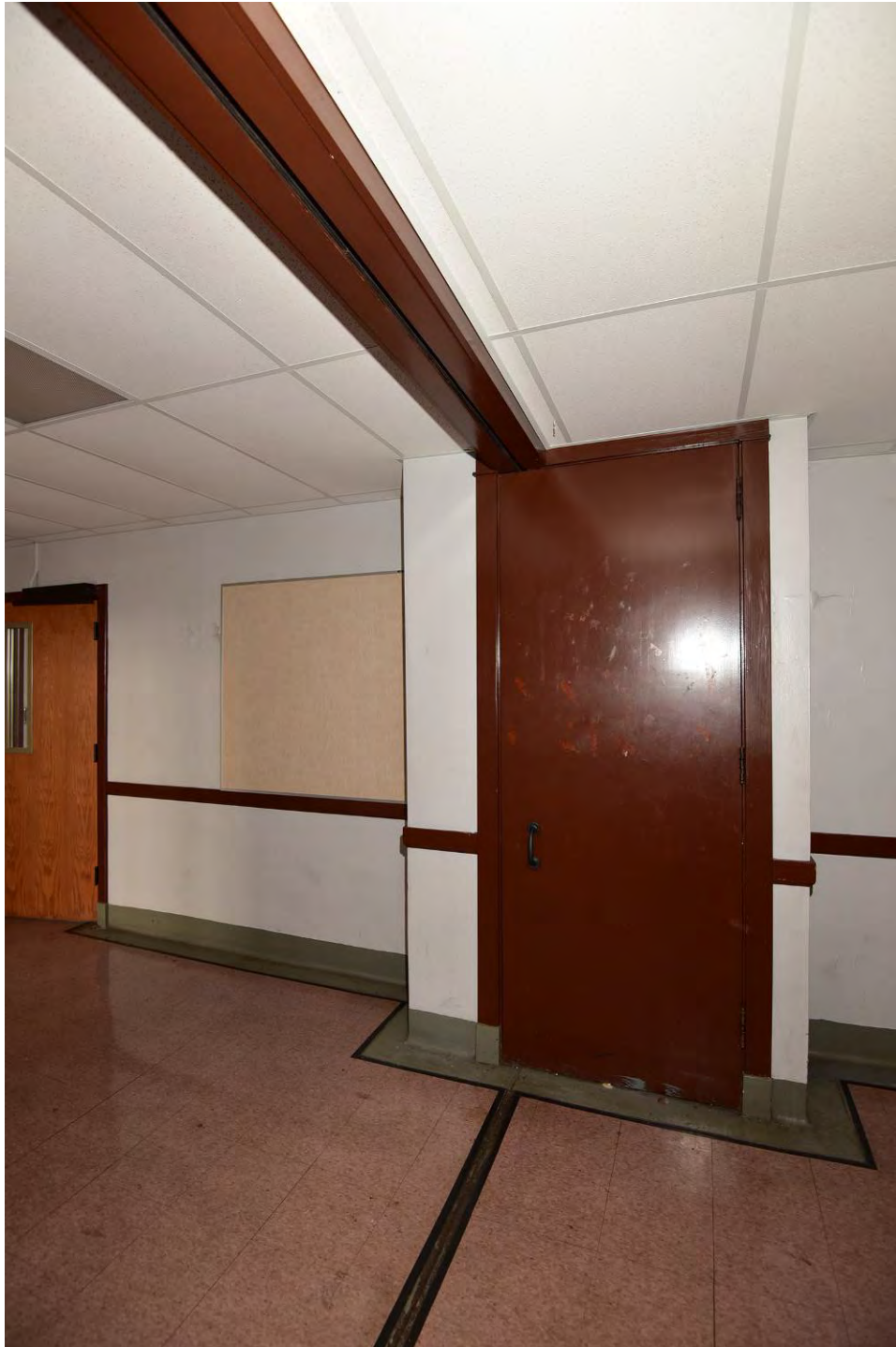
Figure 14. Seam between building campaigns. Source: Brad Finch, 2017.
