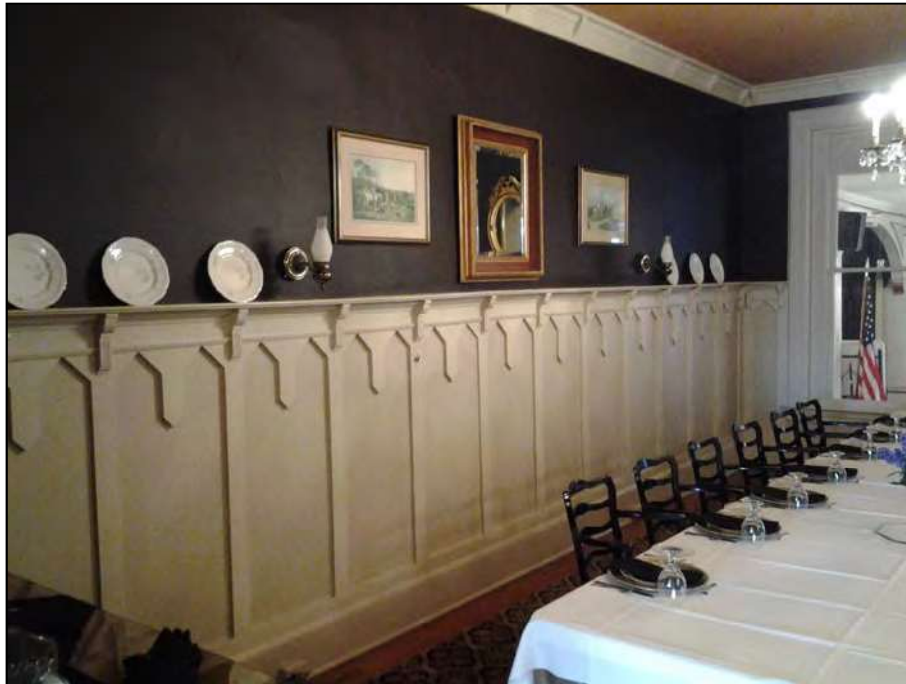
Figure F21. Wainscoting and plate rail in Mirror Room/Black Room. Overlooking garden/ballroom. Camera pointed southwest.
