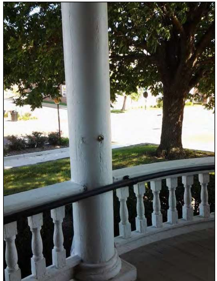
Figure F11. Front porch column with buzzer button for calling attendant – no longer functional. Camera pointed southeast.
