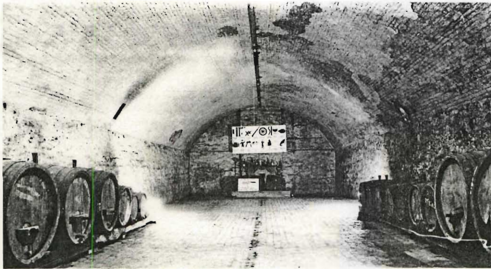
9-1. Wine cellar, Mt. Pleasant Wine Company, Augusta, St. Charles County, constructed 1865-1870. The brick barrel vault was supported by stone walls; the floor was paved with brick.
