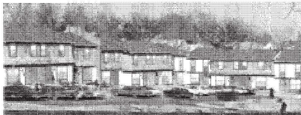
1960s Multi-Family Townhouse (Row House) Complex Kansas City (Missouri) Public Library, Special Collections
