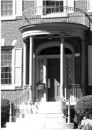
Image J Entrance Portico.
