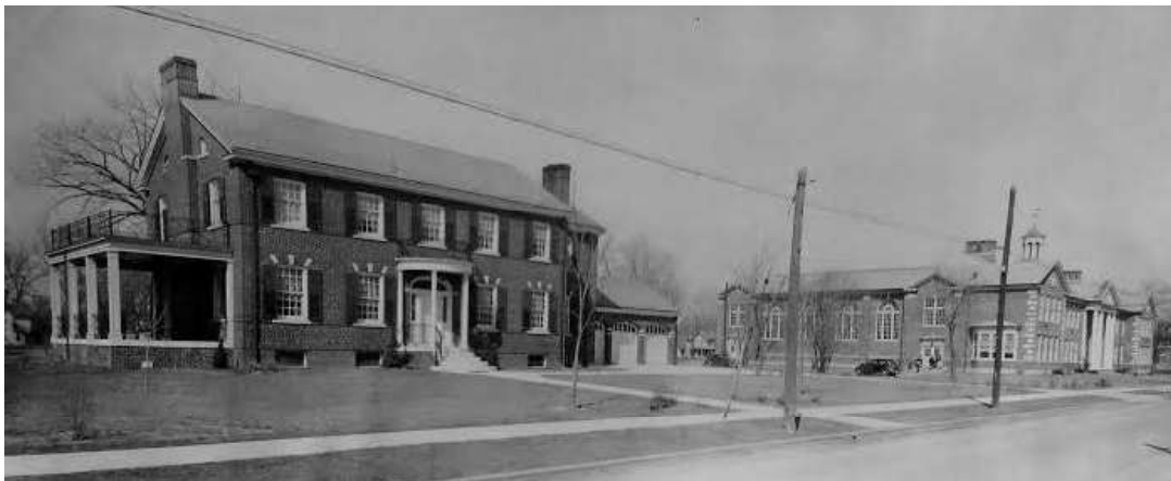
Image BB Laughlin House and Greenwood Elementary School (built 1934-1935. Extant), intersection of Halliburton St. and Normal Ave., circa 1938. (Adair County Historical Society).
