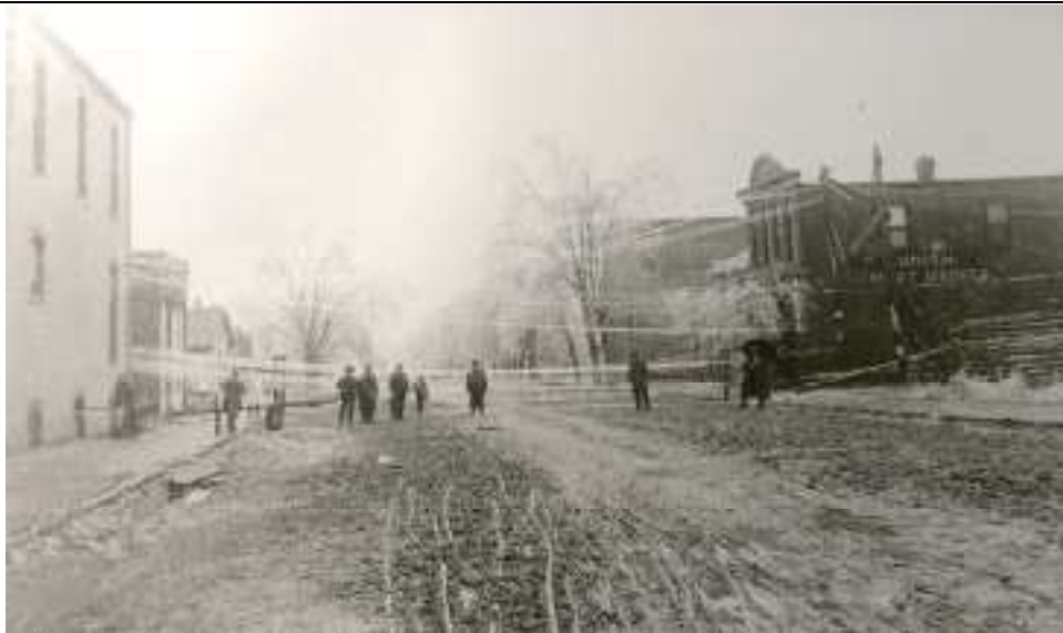
Image C: North Franklin Street after the sleet storm of 3 January 1897. Ivie's Hotel, 102 West Harrison Street, is on the far left and the original facade of the Union Meat Market, 210 North Franklin Street, can be seen on the right.
