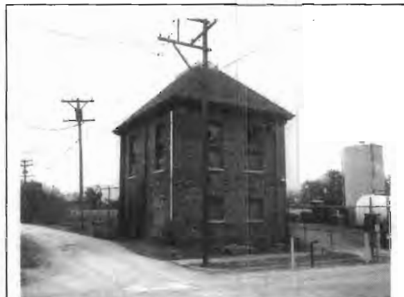
Waterworks Building at 22 nd Street and Murphy Avenue
