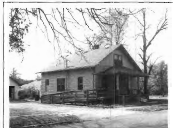
Early Twentieth Century Gable Front House, Bungalow Plan, Rusticated Concrete Masonry Unit Construction, Joplin, Missouri Sally Schwenk Associates, Inc
