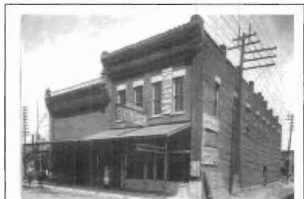
Late Nineteenth Century Vernacular One-Part Commercial Block (left) and Two-Part Commercial Block (right) Joplin Missouri The House that Jack Built Joplin Public Library
