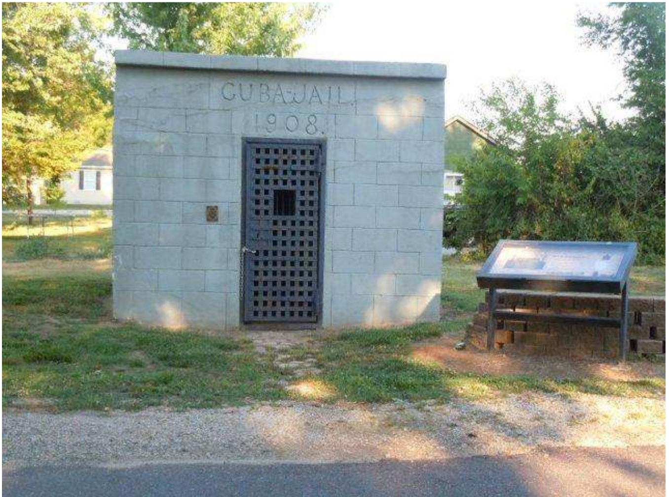
Fig. 11 The 1908 Cuba Jail is the earliest extant building built by the municipality. [photo by Marilyn Stewart]
