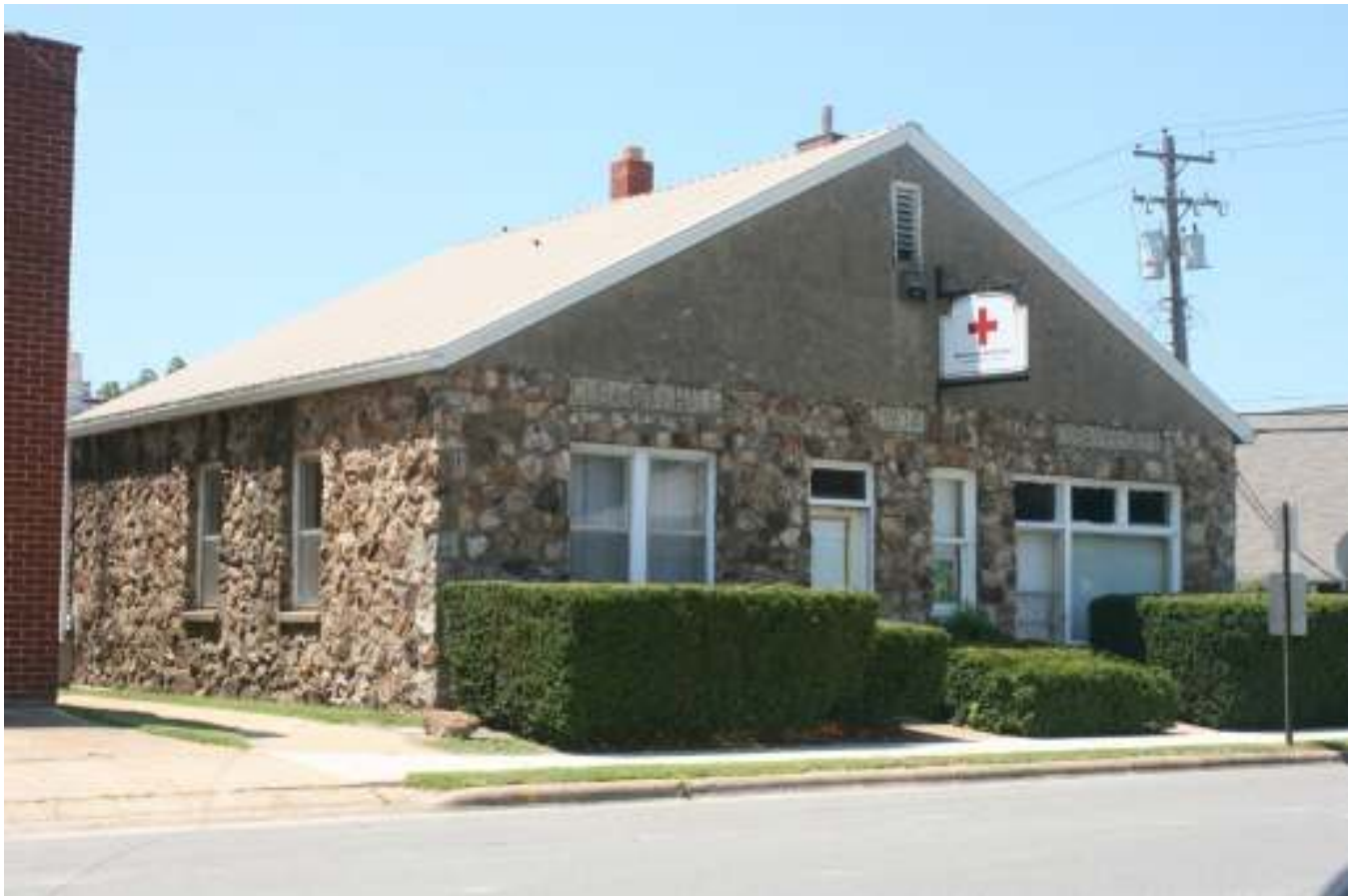
Fig.9 The former Cuba City Hall/Fire Department was built in 1934 with New Deal employment public works funding. It is characteristic of the tradition of stone building which developed in Cuba during this time.
