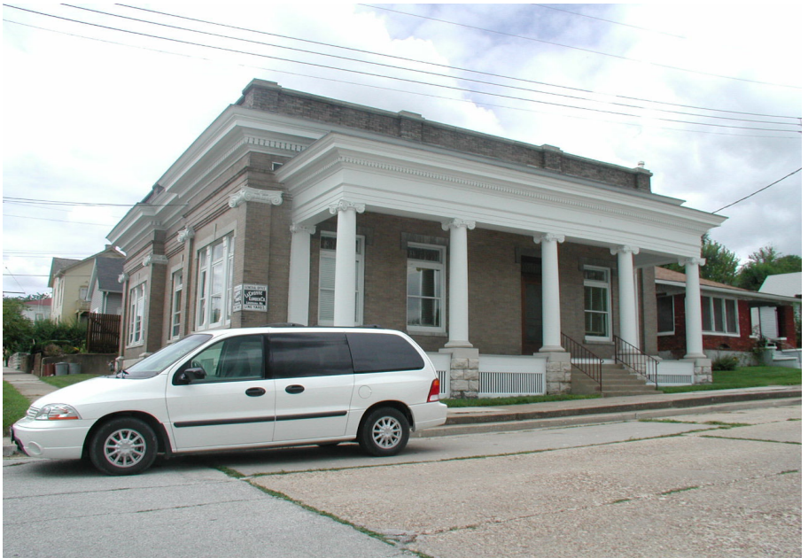
Figure Eighteen. LaCrosse Lumber Company General Offices, 2004.
