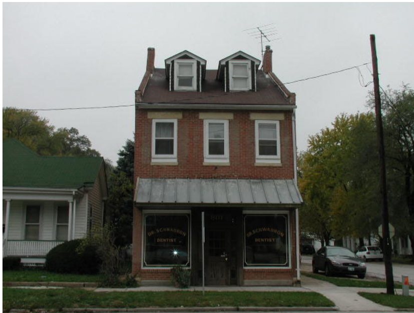
Figure Seven. William Kuhlman Building, 801 Georgia Street, 2004
