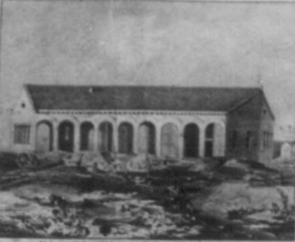
St Louis & Iron Mountain Railroad Work - Shop.
