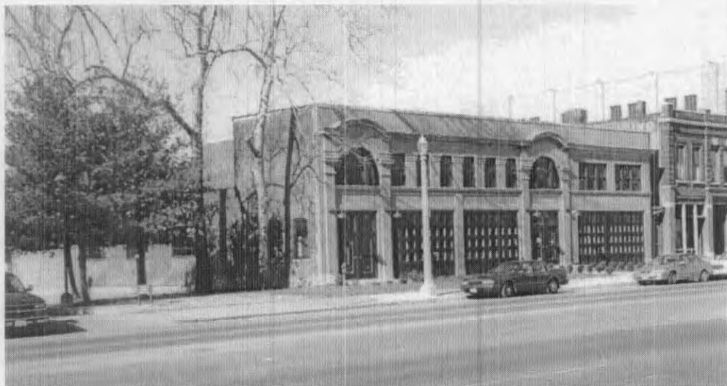
Service Garage 2337-2345 S. Grand
