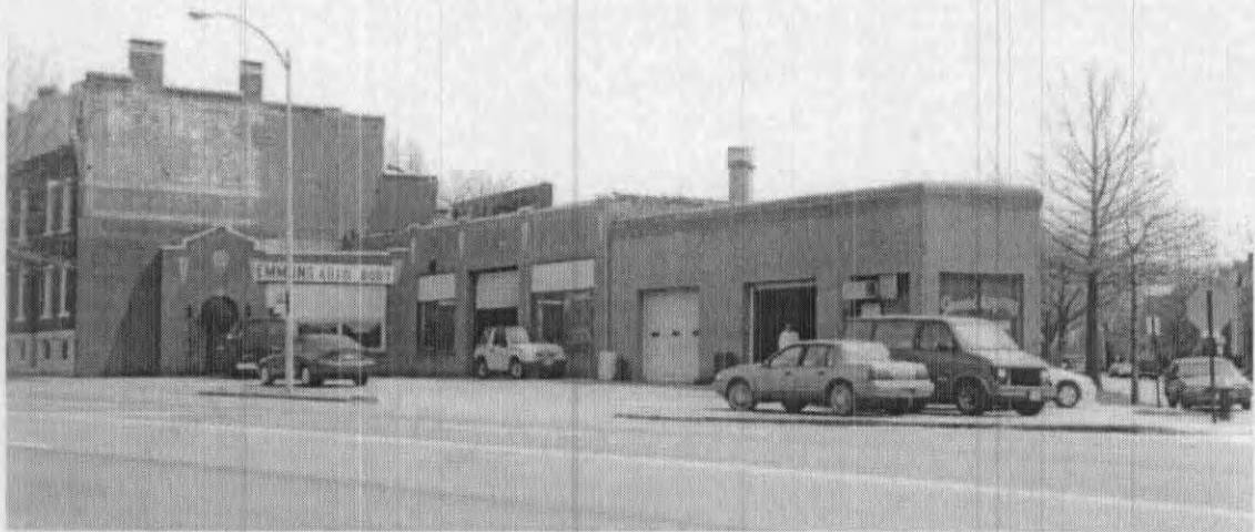
Service Garage 2230 Gravois
