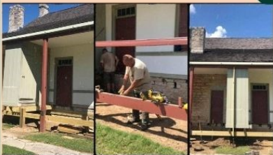
New Back Porch on Felix Valle house 2021
