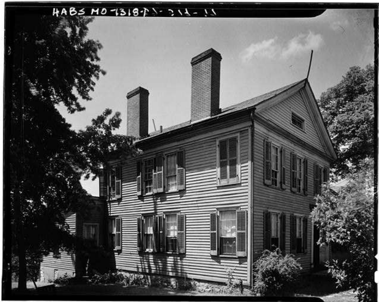
Figure 12: Frizel-Welling House, Jackson, Cape Girardeau, MO Historic American Buildings Survey (Library of Congress), photo c. 1937.
